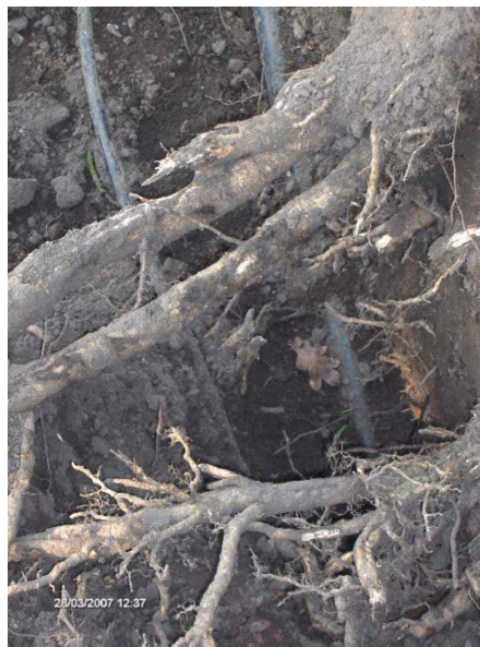
Typical root damage caused by excavation works
