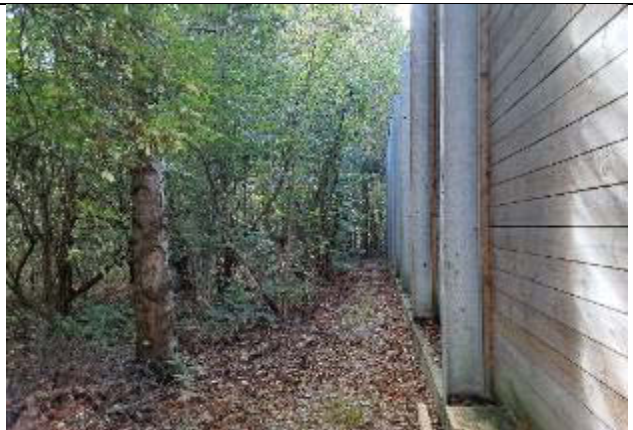
Photograph 19: Northern Cable route- Acoustic fence, adjacent 1m unsealed surface and then plantation woodland. The cable will be fixed to the back of the fence.
