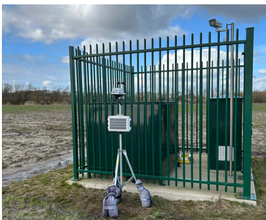
Figure 5.2.6: Lidar and Weather Station
