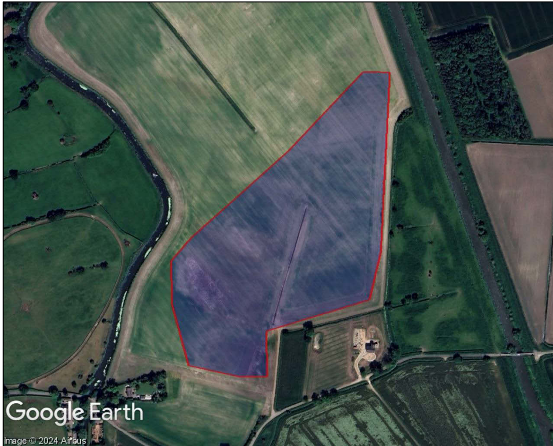
Figure 2 Solar panel area for the proposed development
