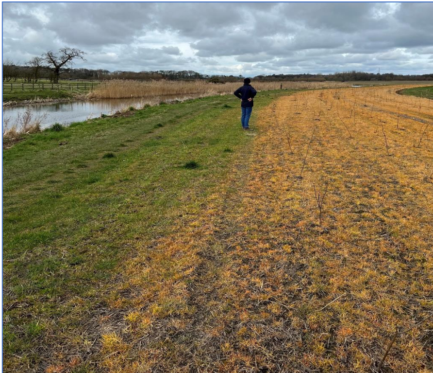
Photograph showing recently planted trees and shrubs, set back 8m from the canal side.
